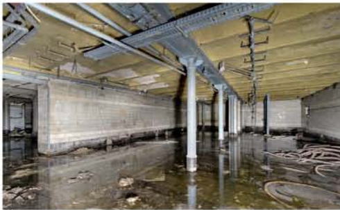
Kesselhaus Keller. © Denny Müller
