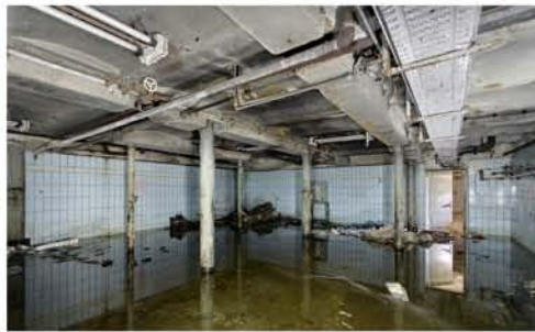
Kesselhaus Keller. © Denny Müller
